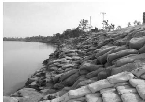
Fig. 5 Sandbags on embankment slope
