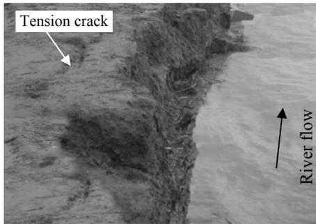
Fig. 7 Riverbank failure in charghat area
