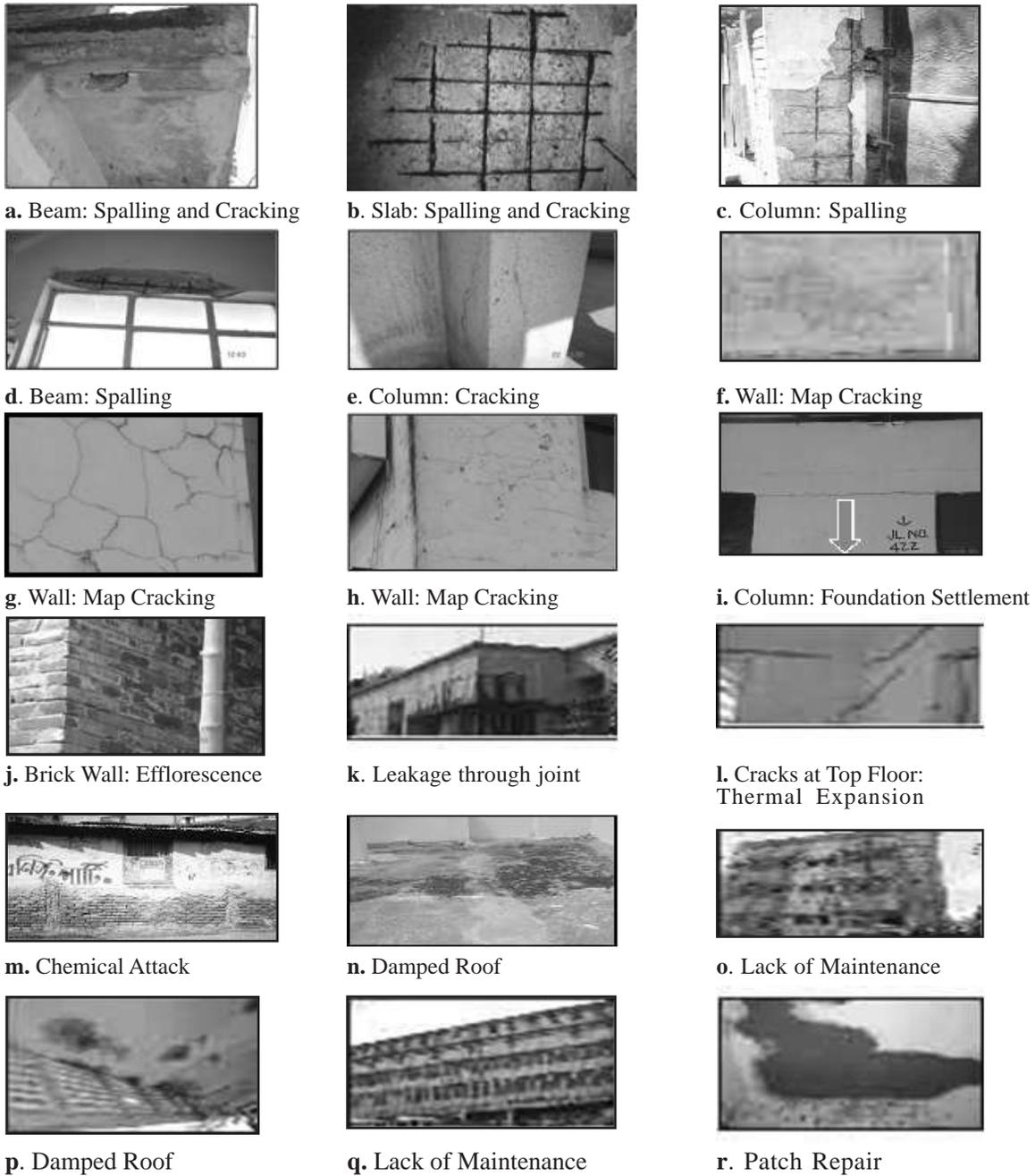
**Figure 2.1** Photographs of some typical types of deterioration observed in concrete structures in Bangladesh.
